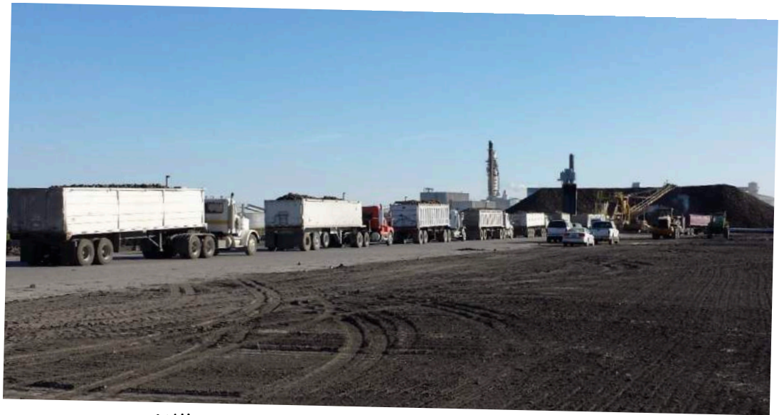
Hillsboro Beet Plant - North Piling Station
